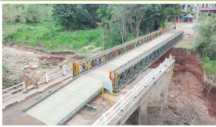
Kandy-Ragala Road (21km)
