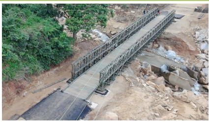
Kandy-Ragala Road (18km)
